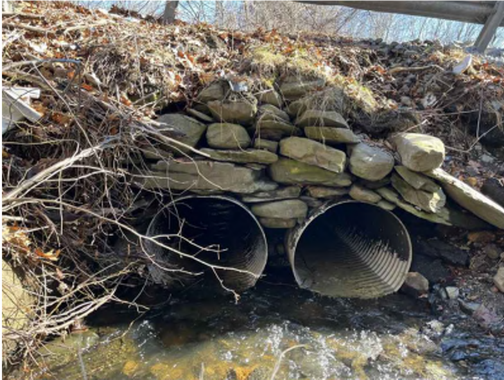
Photo 1: West elevation displaying masonry headwall and barrels #1 and #2.
