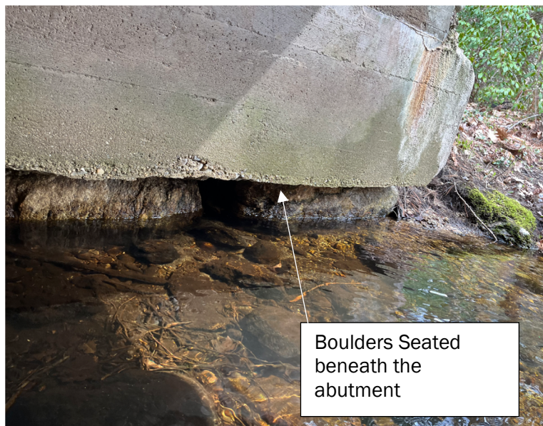
Figure 2-8 L-17-029 North abutment
