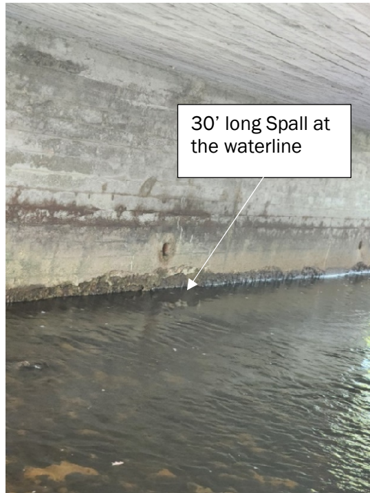
Figure 1-5 L-17-025 South Abutment
