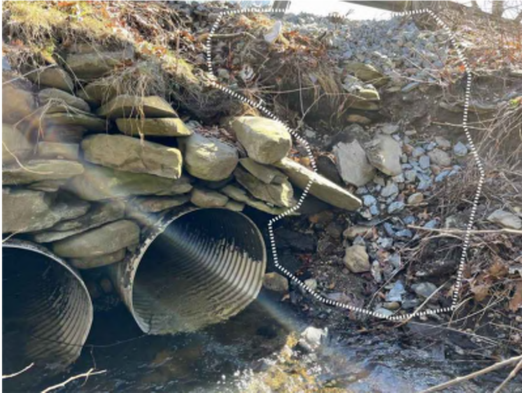
Photo 3: West elevation, South embankment displaying added riprap and erosion.
