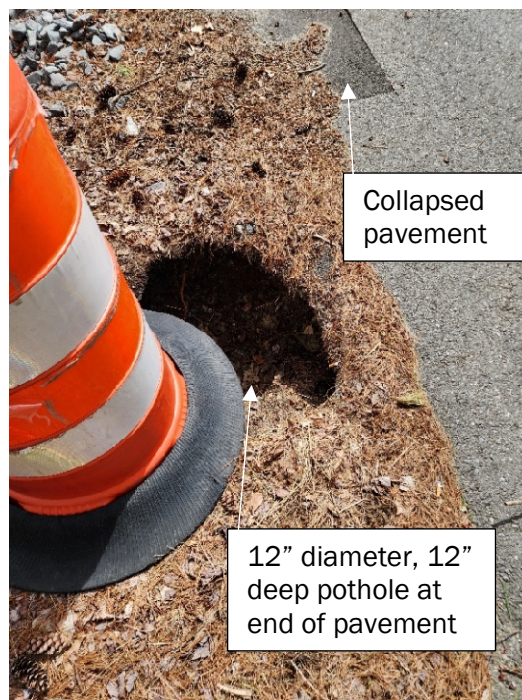
Figure 5-2 L-17-030 Northwest Edge of Wearing Surface
