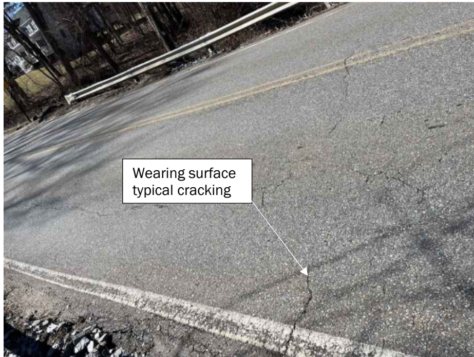
Figure 3-1 L-17-014 Wearing Surface
