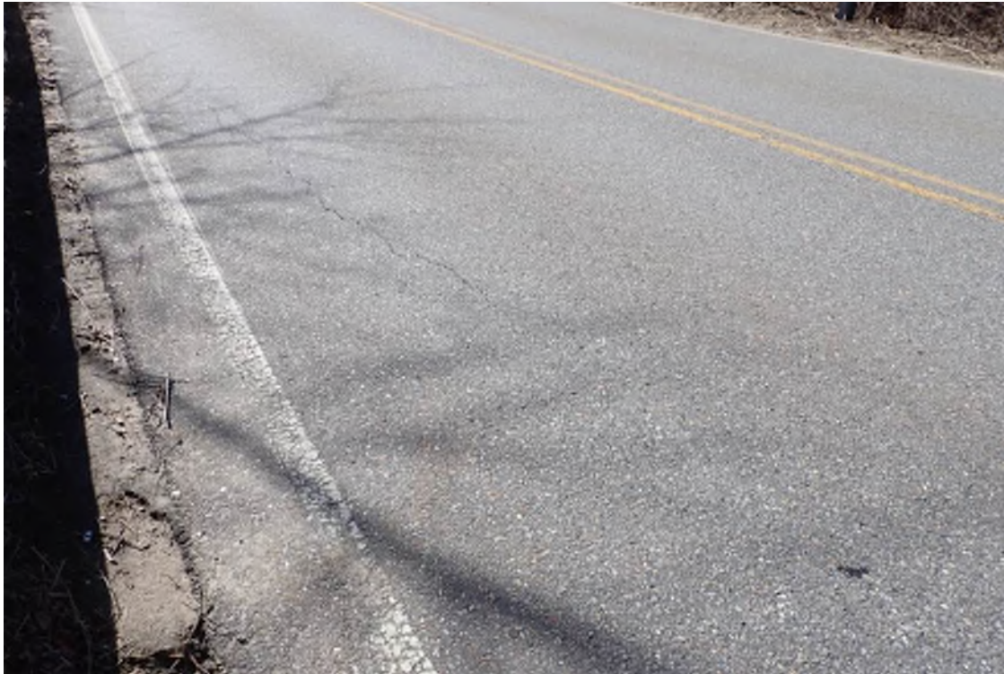
Photo 1: Cracking in the northbound lane.
