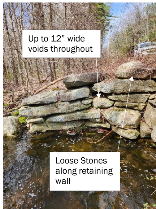
Figure 5-4 L-17-030 Northeast Wingwall
