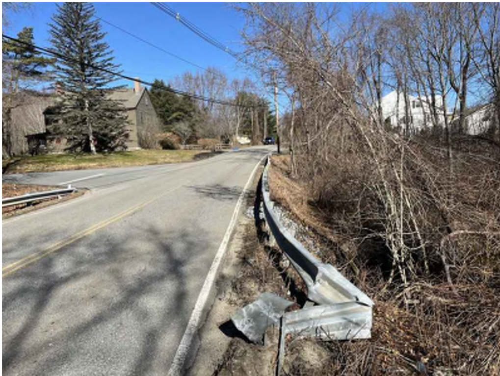
Photo 6: East rail collision damage.
