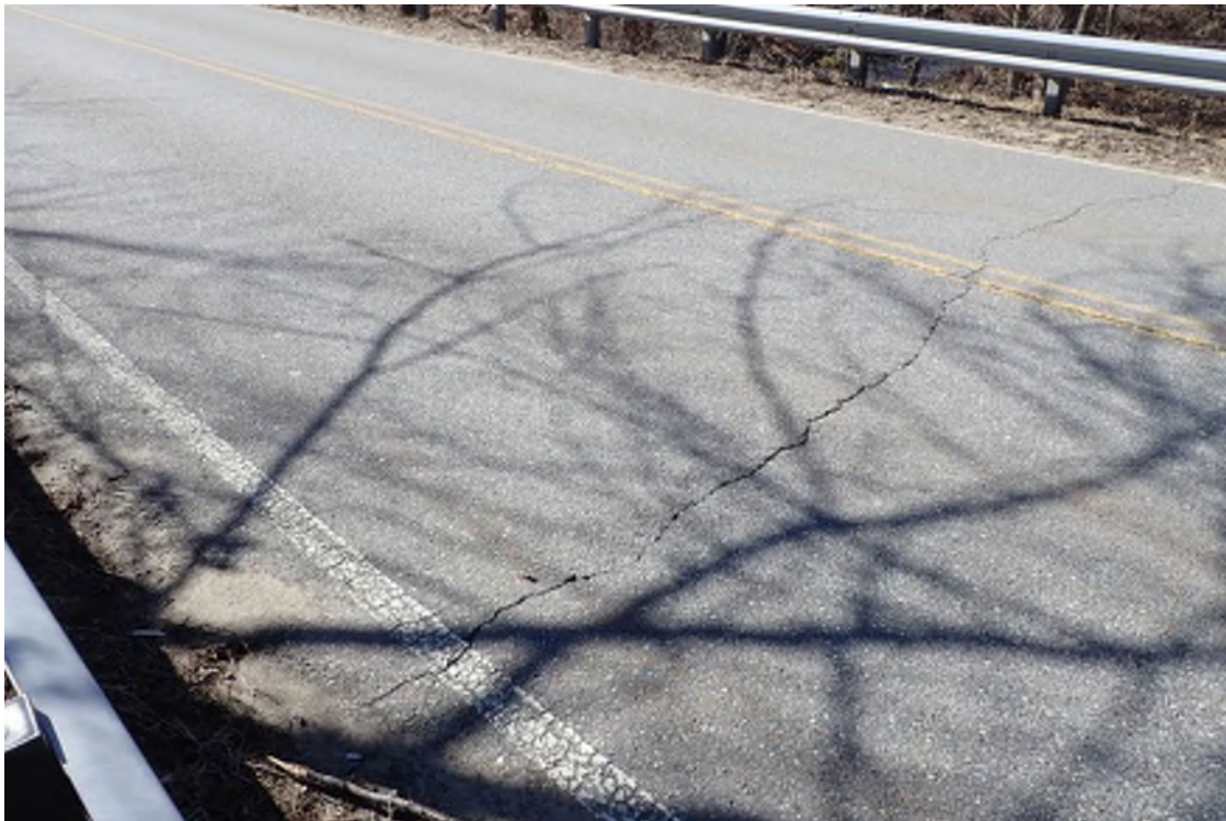
Photo 2: Approach pavement cracking.
