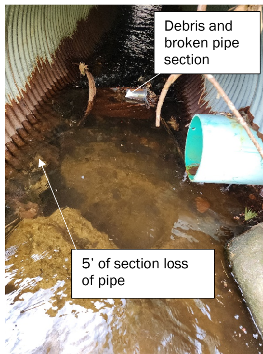
Figure 5-6 L-17-030 North Elevation drainage pipe
