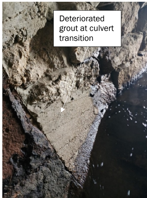
Figure 4-3 L-17-031 Grout at Culvert Transition
