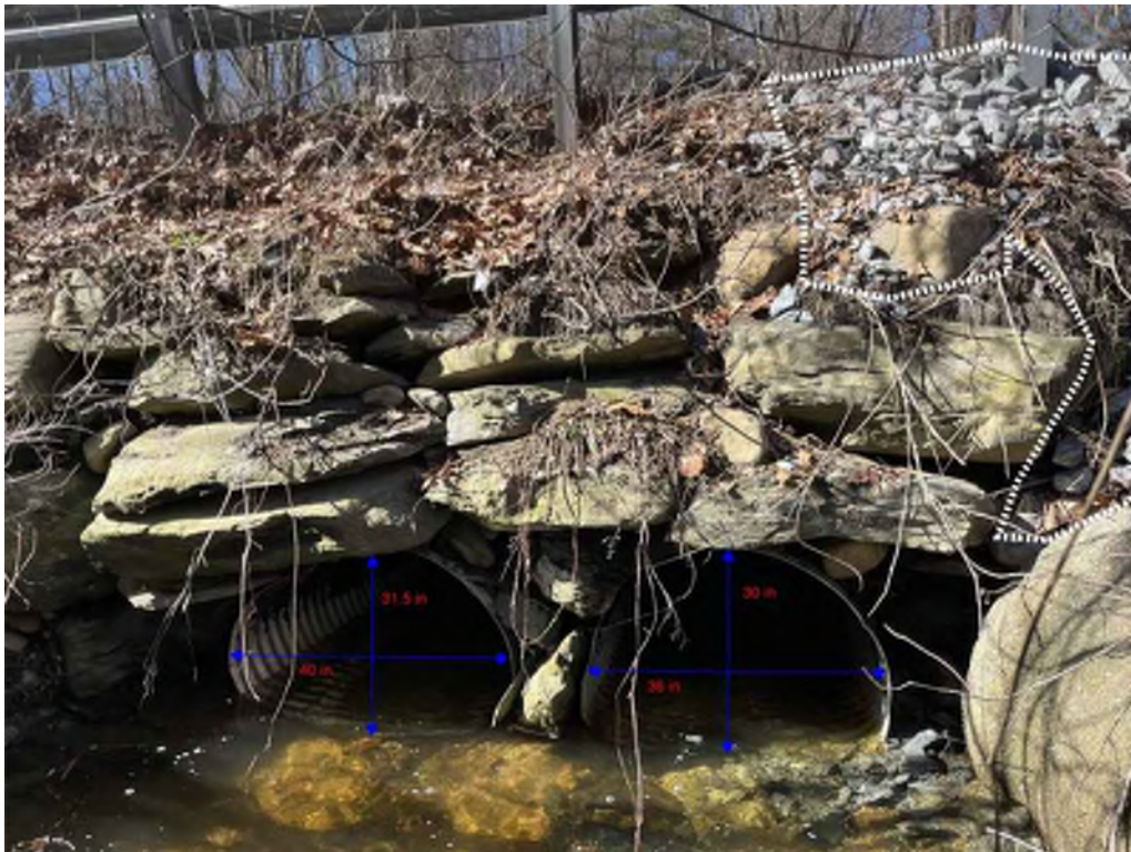
Photo 2: East elevation displaying deformed barrels and added embankment.
