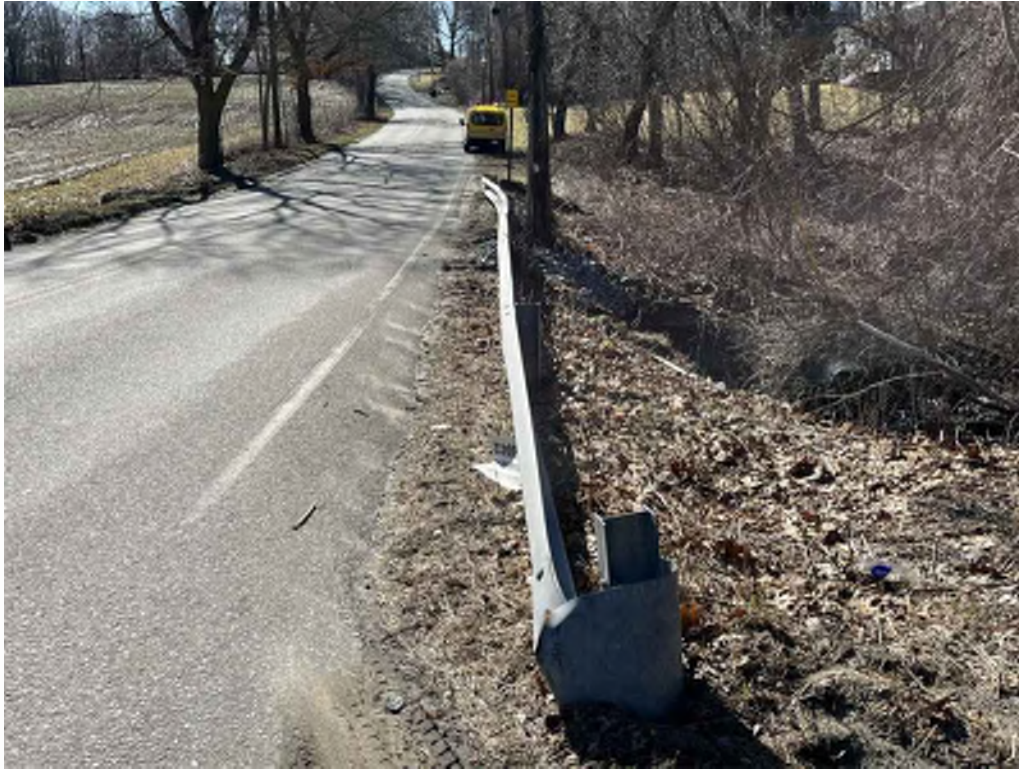
Photo 5: West rail collision damage.
