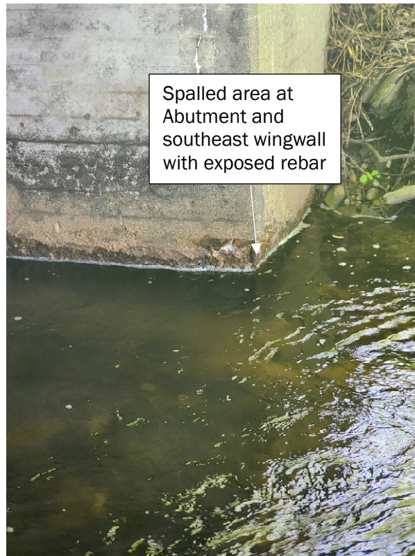
Figure 1-7 L-17-025 south breastwall and southeast wingwall
