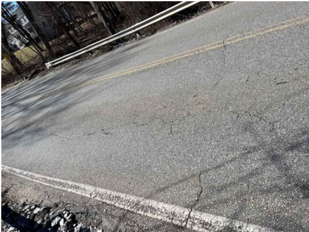
Photo 4: Wearing surface typical cracking.
