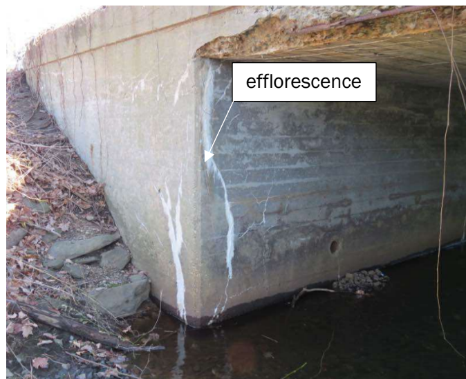
Figure 1-8 L-17-025 Northwest wingwall
