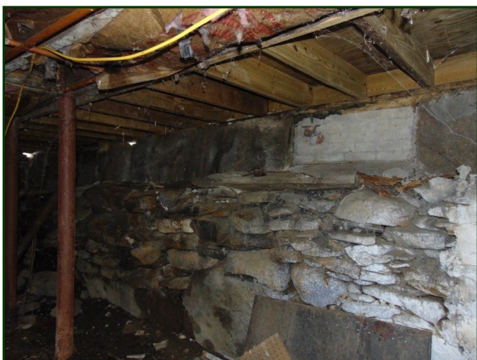
Photo #41: Stone foundation exposed in the basement.
