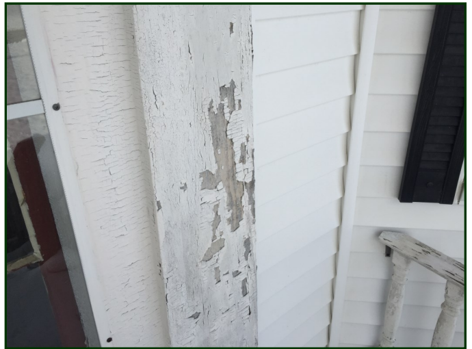
Photo #4: Photograph depicts general view of peeling/flaking paint on exterior trim
