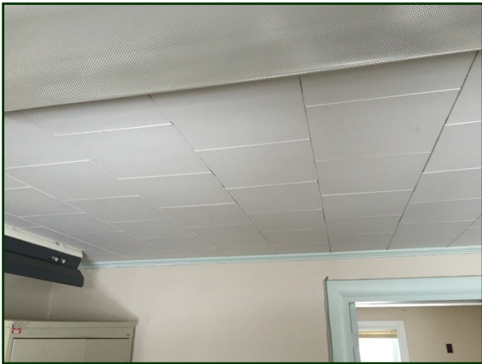
Photo #57: Photograph depicts general view of the 1'x 1' Ceiling Tile within the 2nd Floor Office Area
