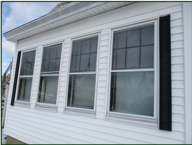
Photo #9: Vinyl clapboard siding and double hung wood windows
