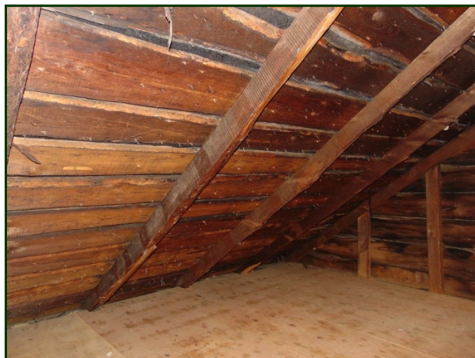
Photo #48: View of typical roof framing.
