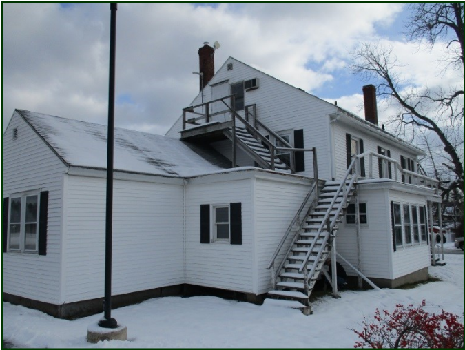
Photo #4: View from northwest corner of building. Note wooden fire escape
