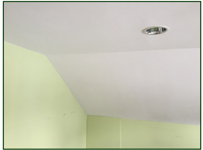
Photo #56: Photograph depicts general view of the Wall-board Walls and Ceiling within the 3rd Floor
