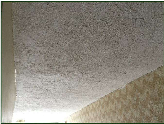
Photo #55: Photograph depicts general view of the Textured Ceiling with the 2nd Floor Hallway
