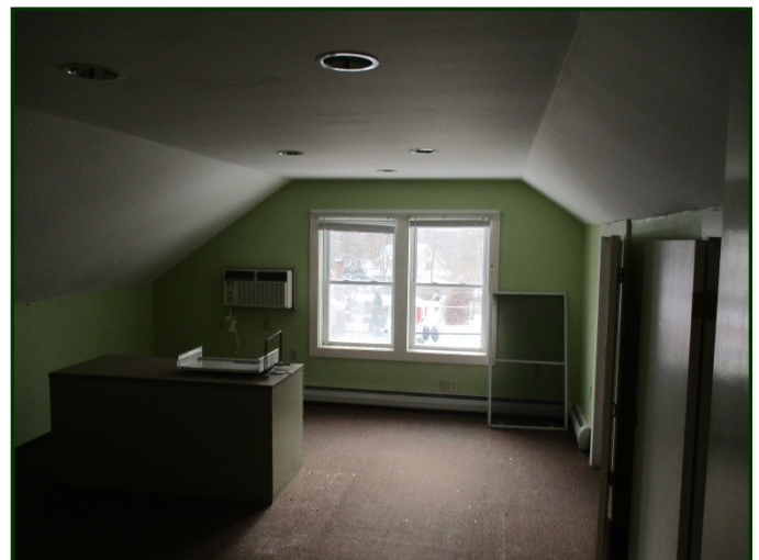
Photo #24: Finished attic level with carpet floor and painted gypsum board ceiling and walls
