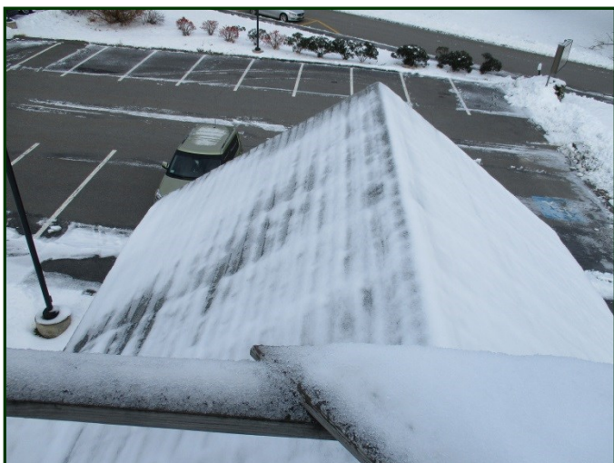
Photo #13: Asphalt composition roofing shingles. Note asphalt-paved parking lot beyond (north side of site)
