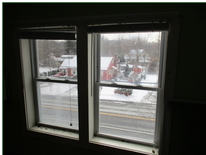
Photo #16: Newer (circa 1998) double hung vinyl windows with insulated glazing at upper floor level
