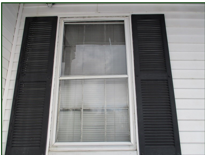
Photo #15: Original (circa 1935) double hung wood windows with non-insulated glazing on the first floor level
