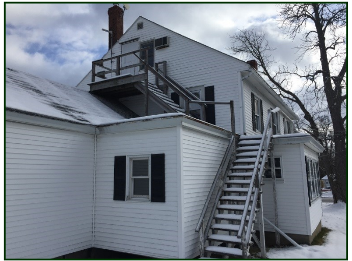
Photo #50: Photograph depicts general view of the backside of the Site Building
