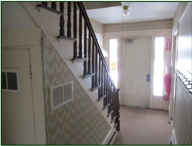
Photo #19: Main front entrance. Note carpet floor, wall covering and painted plaster ceiling and wood trim
