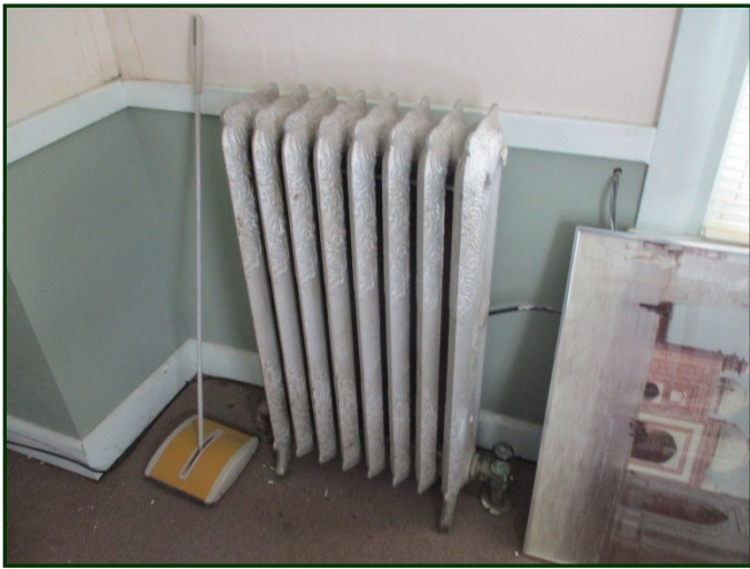
Photo #31: Cast iron radiator
