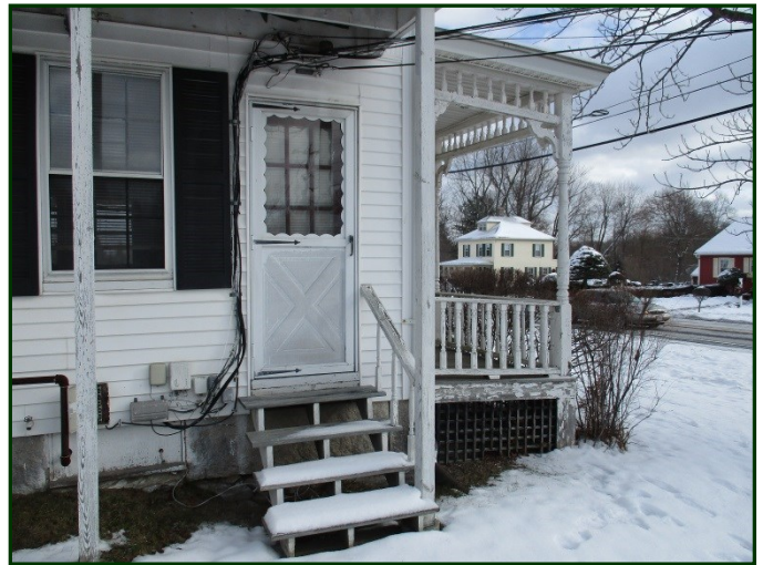
Photo #10: Secondary entrance at southwest corner of building
