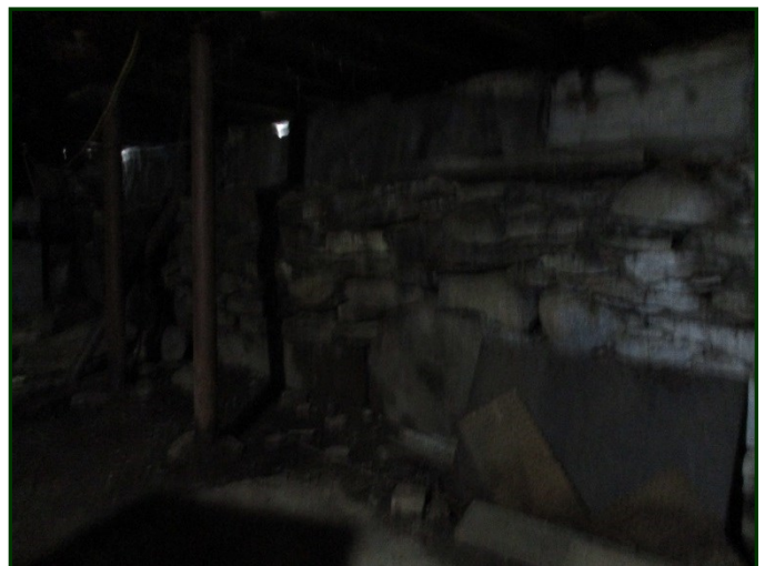
Photo #30: Stacked stone foundation. Note daylight at top of foundation wall
