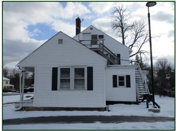
Photo #8: North elevation
