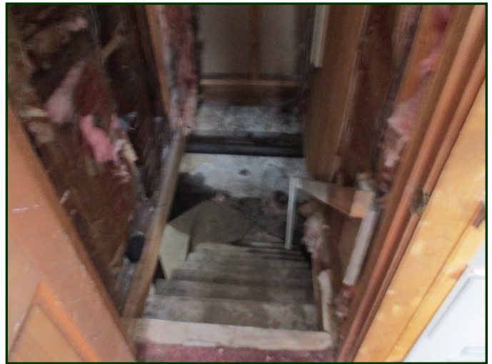
Photo #28: Stairway from first floor to basement
