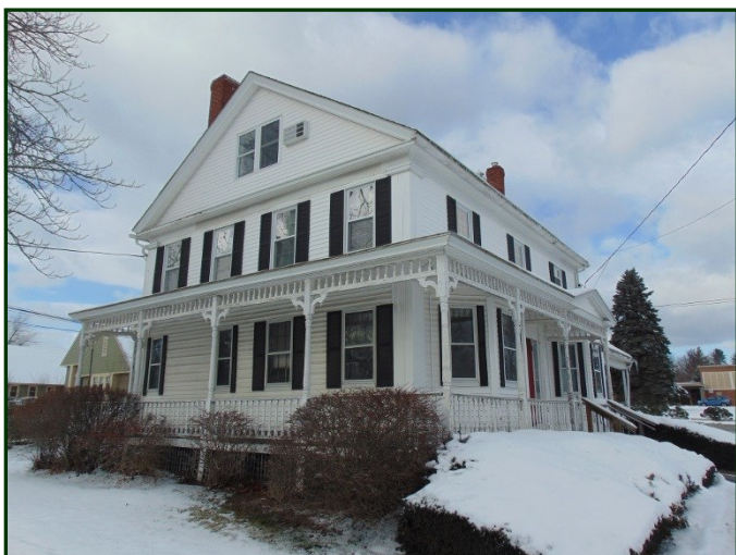
Photo #37: South (front) elevation of Brooks House. Note wrap-around porch.
