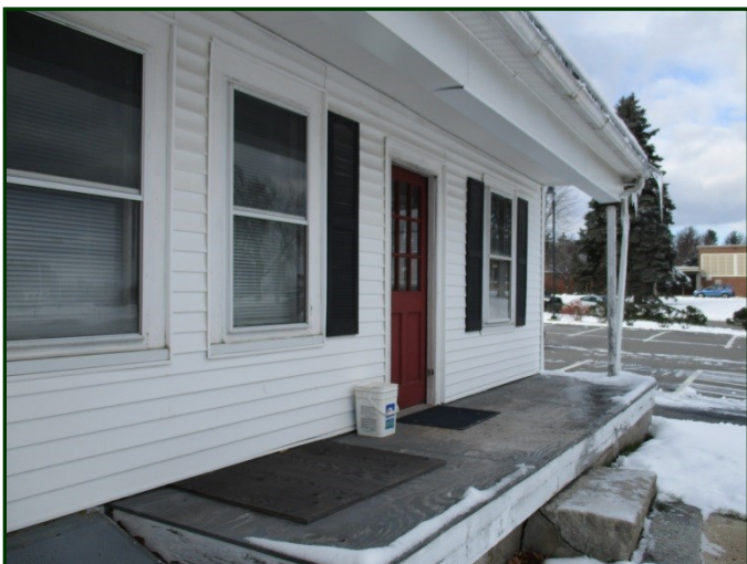
Photo #11: Secondary entrance at northeast corner of building
