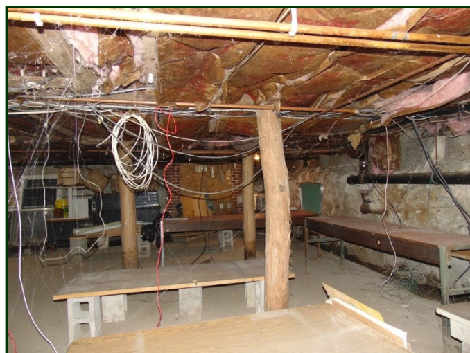
Photo #42: Typical round wood post supporting ground floor.
