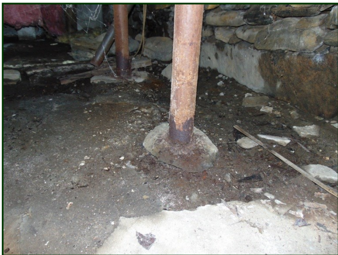
Photo #43: Steel posts supporting the north one-story wing of the Brooks House.
