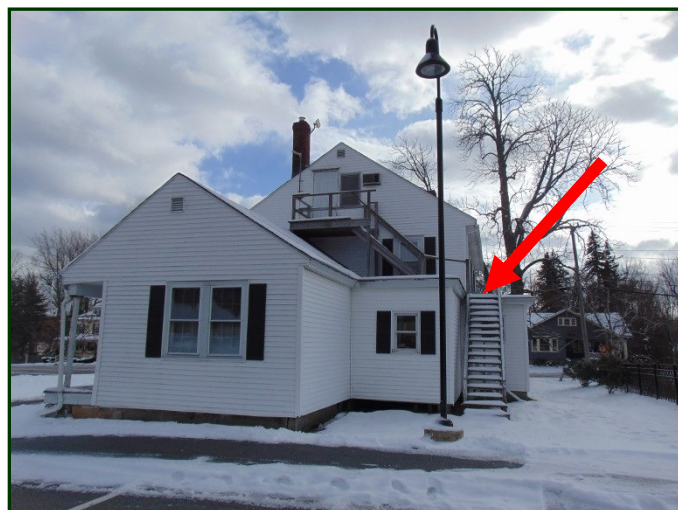
Photo #40: North (rear) elevation of Brooks House. Note 2nd floor fire escape.
