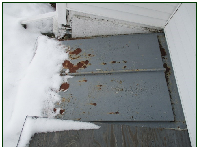
Photo #12: Painted steel bulkhead at east elevation
