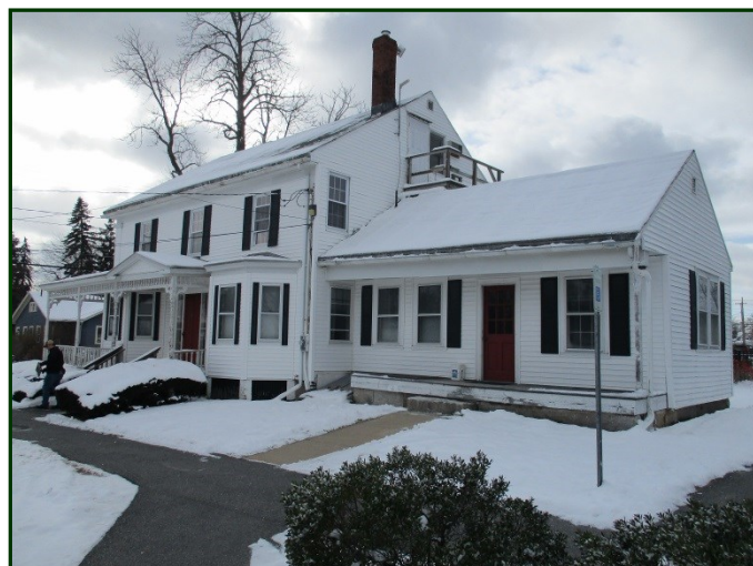
Photo #14: View from northeast corner of building
