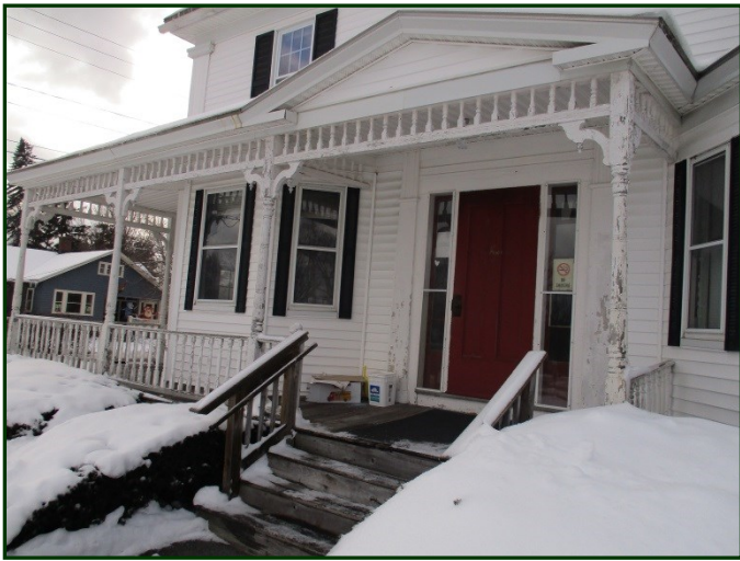
Photo #7: Main front entrance at east elevation
