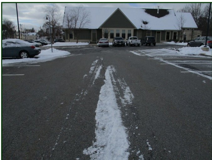
Photo #17: Asphalt-paved parking lot on north side of site
