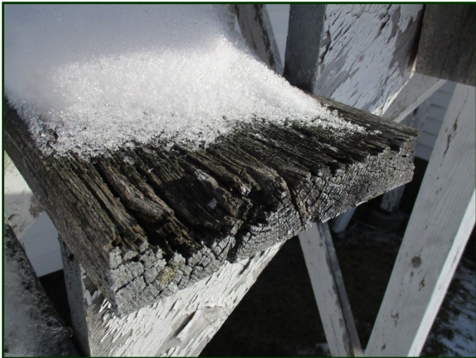
Photo #5: View of deteriorated wood at fire escape
