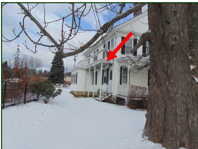
Photo #39: West (side) elevation of Brooks House. Note 2nd floor fire escape (indicated by arrow).
