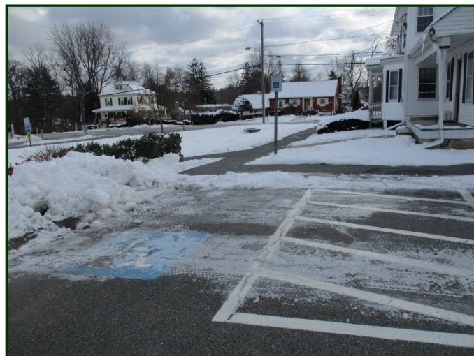
Photo #18: Accessible parking space adjacent to building entrance
