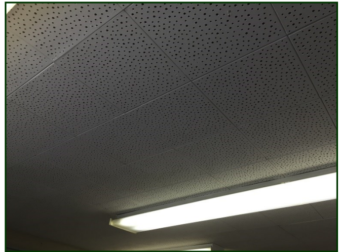
Photo #58: Photograph depicts general view of the 1'x 1' Ceiling Tile within the 1st Floor Office Area
