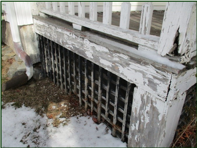
Photo #6: View of deteriorated wood at front porch
