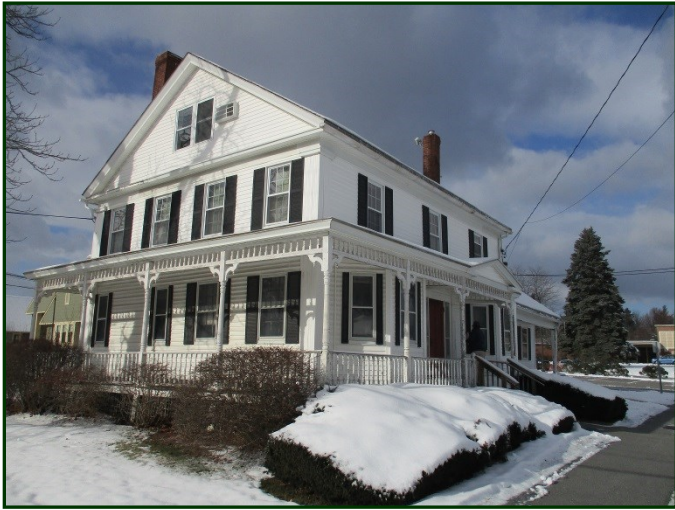
Photo #1: Overview from southeast corner of building
